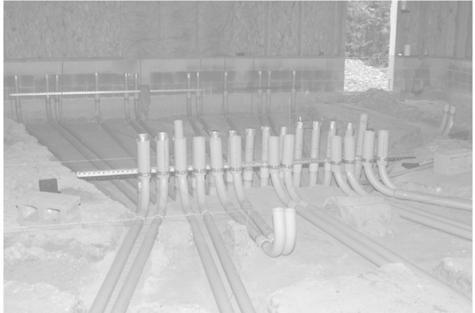
Figure 6.3 1 Low-voltage conduits.
