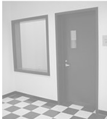
Figure 5.4 1 Overly Door Co. window.
