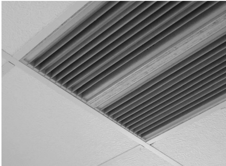
Figure 9.20 PI 324 Quadratic Residue Diffusor in ceiling grid.
