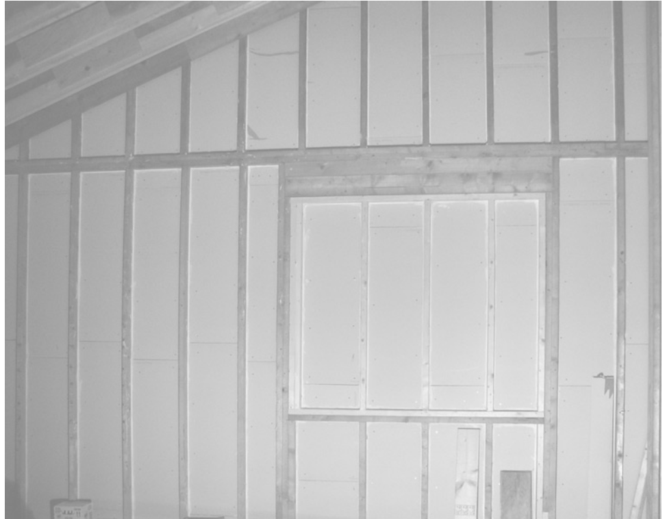
Figure 10.18 Exterior wall isolation.
