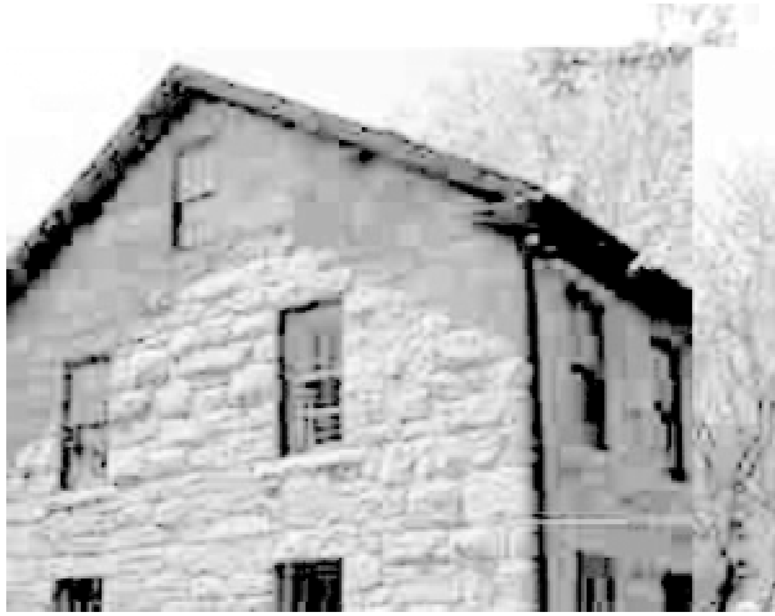
Figure 8-30. Photograph showing a medium level compression
