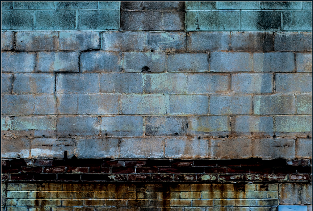
Block and brick wall
