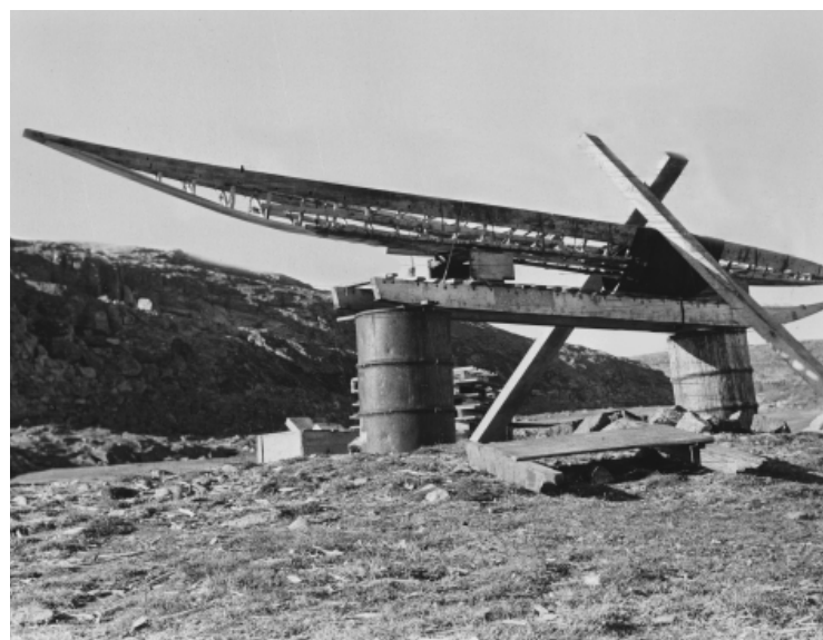
Figure 8.8 —Rebuilt framework of Ainalik's kayak raised above the reach of dogs, who would eat the sealskin lashings. The paqaq , or cockpit hoop, will be added later. Photographer E. Arima, 1960. © Canadian Museum of Civilization, no. J16403.
